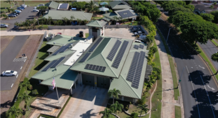
New 56 kilowatt solar photovoltaic system on the roof of the 'Ewa Beach Fire Station. (Photo Credit: Department of Design and Construction)
