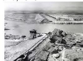
Banqiao dam failure; China, 1975
