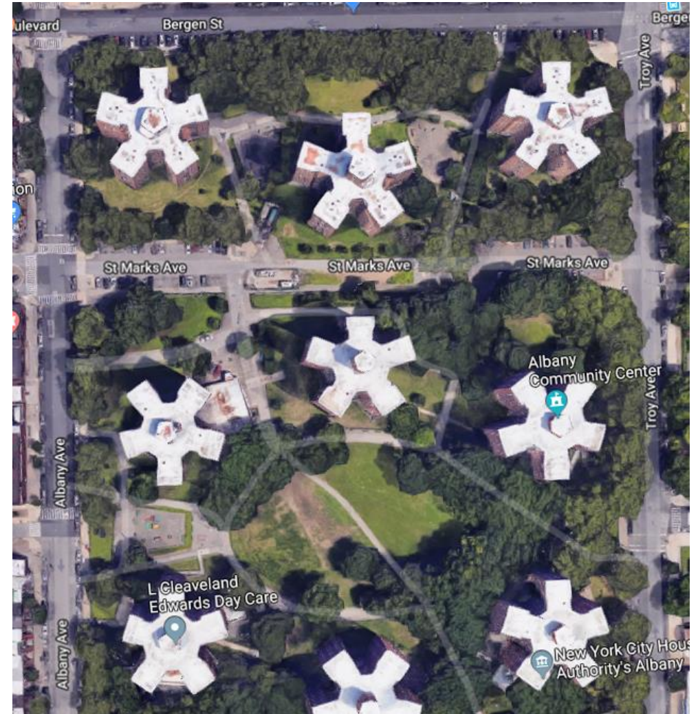
NYCHA – Albany Houses after roof coating in 2018
